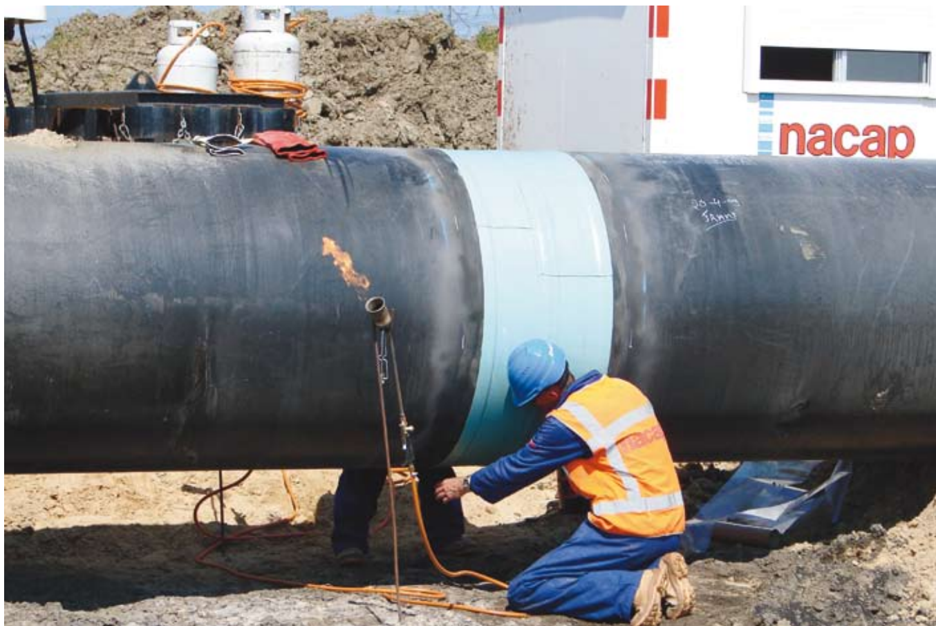
Figure 2. Application of shrinkable sleeve over Stopaq's Wrappingband CZH.
