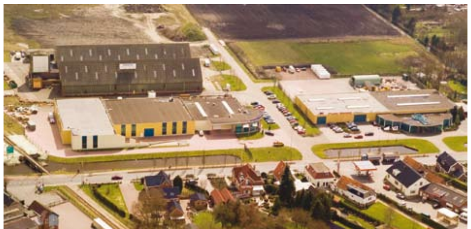
Figure 4. Stopaq, Stads kanaal, The Netherlands.
